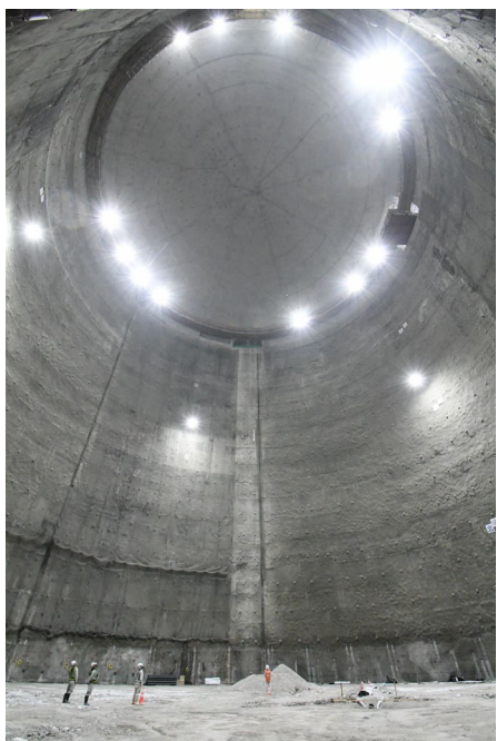
Cavern excavation (~2025, Jul.)
