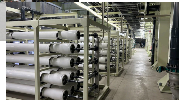
Pure-water system: under construction (@ 2026, Apr./May.)
